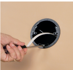
2 Pull cable and tighten mounting wing screws to hold bracket secure.
