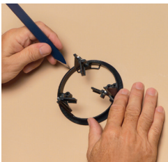
1 Bracket is template for opening.
