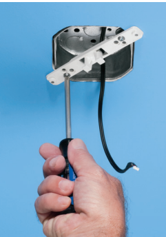
1 Attach SC5 bracket to box.
