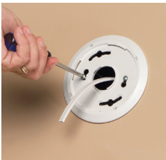
3 Install mounting plate per manufacturer's instructions.
