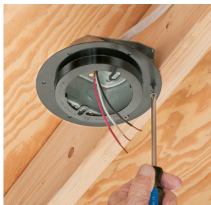
...through the device holes or flashed-over holes to hold it in place during drywall installation.
