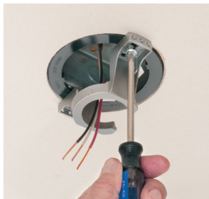
After drywall installation, install fixture or fan bracket per manufacturer's instructions.
