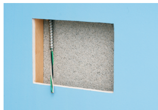
1 Determine box location. Cut opening in wall.
