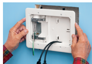
2 Pull metal conduit through opening. Insert box.
