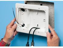
**4** Install trim plate. Pull cable through connector. To install box in hole tighten wing screws (see 3).
