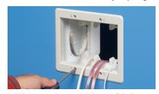
3 Tighten mounting wing screws to pull the box securely against the wall.
