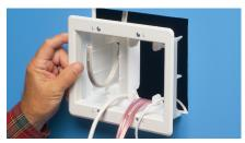
2 Cut drywall. Attach trim plate to box. Pull wire/cables. Install box assembly in opening.
