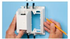
1 Use enclosure (without trim plate) as a template for opening. Cut hole.
