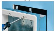
Cut hole using enclosure, without trim plate, as a template. (Mounting wings hold box in wall.)
