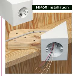
Cut a 2x8 approximately 18" long. Install FB450 on 2x8 allowing it to extend 8 to 10" past the box. Keep bottom of box level, short side of box touching angled rafter. Nail or screw assembly to rafter.
