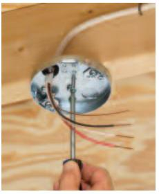
3 Pull NM cable through installed NM cable connector – or where metal raceway is required by code, remove NM cable connector and install appropriate fitting.
