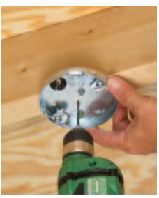
2 Remove mud cover. Remove four box installation screws (shipped in place). Use these screws to install box to joist through pre-drilled holes.
