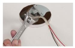
Use a wrench to tighten hex bar, embedding the points and securing the brackets between the joists.
