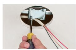
Loosen sled screws. Slide to along bracket to access the hex bar. \*\*There is no need to remove the sled.
