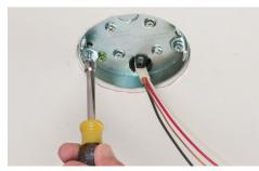
Center box in hole. Tighten sled to hex. Pull cable through NM cable connector and remount box to the bracket. Attach fan/fixture bracket to box using the supplied screws.
