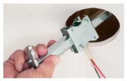
Cut a 4-3/8" diameter hole. Remove pan box from sled. Insert mounting bracket into hole, positioning it between the joists with 'feet' resting on the ceiling.
