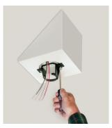
Installing fan bracket on installed box on sloped ceiling
