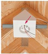
Push cable through installed NM cable connector in box.
