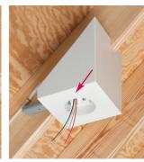
Push cable through installed NM cable connector in box.
