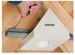
Save time! NO need for a 2x4! Mount steel bracket to angled rafters with short sides of box touching each rafter. Keep bottom of box level. Screw the bracket to the rafters with (4) supplied #10, 1-1/2" wood screws through the pre-drilled screw hole(s) in bracket.
