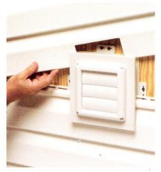
4 Install siding. Overhang on vent flange hides cut ends of siding.
