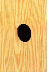
1 Cut hole in substrate with a 4-1/2" hole saw.
