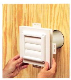
2 Insert vent tube into opening.
