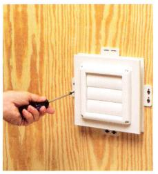
3 Use screws to mount dryer vent to substrate through flanges.
