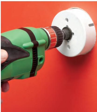
Determine bracket position. Cut opening with a 3.5" hole saw.
