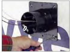
6 Attach the box to the substrate with screws (not provided). At this point it's ready for the installation of the stone or brick.
