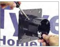
4 ...then secure the box by tightening the four 1/2" screws provided.
