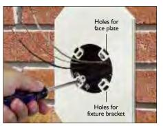
7 After the mortar is dry, attach the face plate to the box with the #8 screws (provided), rotating it so it is perfectly aligned for the fixture installation. Use one set of holes for the face plate, the other set for the fixture bracket.
