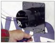
6 Attach the box to the substrate with screws (not provided). At this point it's ready for the installation of the stone or brick.
