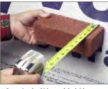
1 Determine the thickness of the brick or stone material, by measuring from the substrate to the front face of the material.
