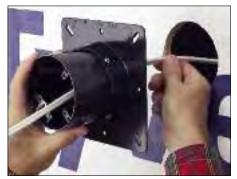
5 Locate the position of the hole, and cut it out with a 4-1/8" hole saw. Pull the cable through the installed NM cable connector.
