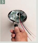
Pull cable through installed NM cable connector. Reattach box, and center it in hole. Attach fan/fixture bracket with supplied screws.
