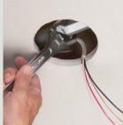
Tighten the hex bar with a wrench to secure bracket between joists. As the hex bar is tightened, bracket ends bite into the joists, holding the unit secure.
