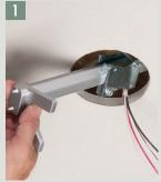
Cut a 4-1/16" diameter hole in ceiling. Remove box from sled and fit mounting bracket into hole. Position bracket between joists, with bracket resting on the ceiling.
