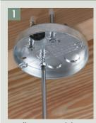
Install FBS405 on joist using shipped in place screw near center of box.
