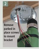
Drill (2) 1/8" diameter holes into joist through the elongated openings on each side of box. Remove the (2) long screws noted above to mount the fan/fixture bracket.
