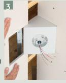
Cut and position drywall to fit around the box. (Note: captive screws in box.) Install fan or fixture per manufacturer's instructions using captive installation screws.
