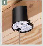
Position box alongside joist. Tightening center screw will mount box to joist.
