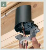
Position mounting bracket over locator posts to assure proper position. Pull wires through KO.
