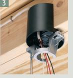
Remove captive bracket installation screws. Use them to mount fan/fixture bracket. (Installation of drywall not shown.)
