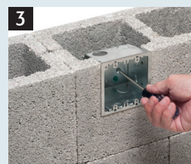
Tighten the screws on the spring clip to pull it securely against the block.
