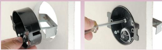
Cut hole in drywall. Insert box and bracket. Box is secured by tightening screws that pull bracket against drywall.
