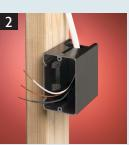
Pull wire through the knockout connector. (Ships with installed NM cable connector.)
