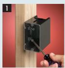
Attach ONE-BOX to wood or steel stud with captive installation screws. If the box is too far forward or back, simply back the screws out and reposition.
