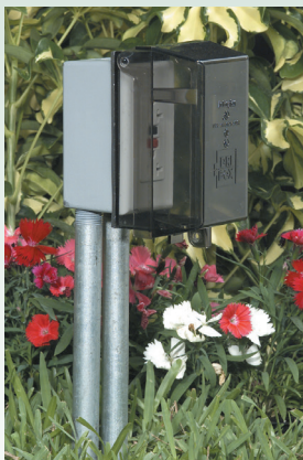
Why install boxes this way...
